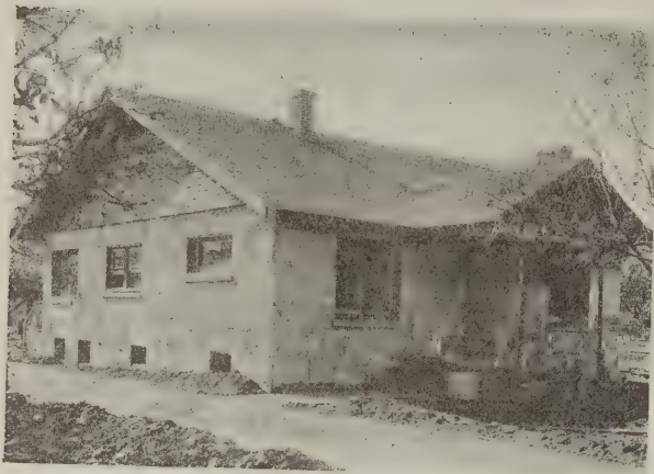
The double walled concrete block bungalow ready for stucco finish
